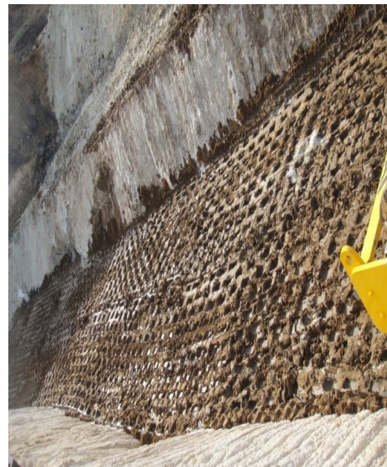
Fig 7.4. Trench filling across the bund section
