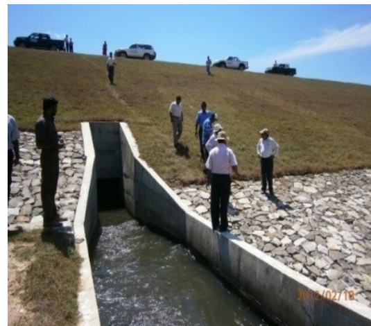
Fig 7.9. Sluice outlet transition and toe area
