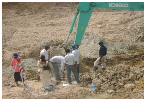
Fig. 6.2. Geological investigation surveys at site
