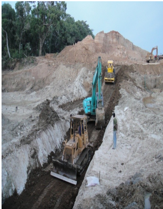
Fig 7.3 Trench filling across the bund section
