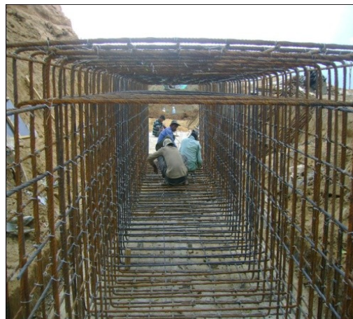
Fig 7.5. Sluce barrel construction
