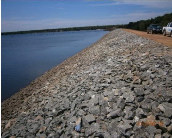
Fig 7.6. Completed u/s embankment
