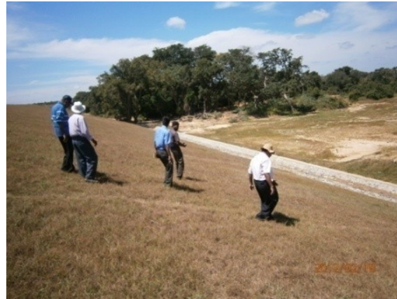
Fig 7.7. Completed d/s embankment
